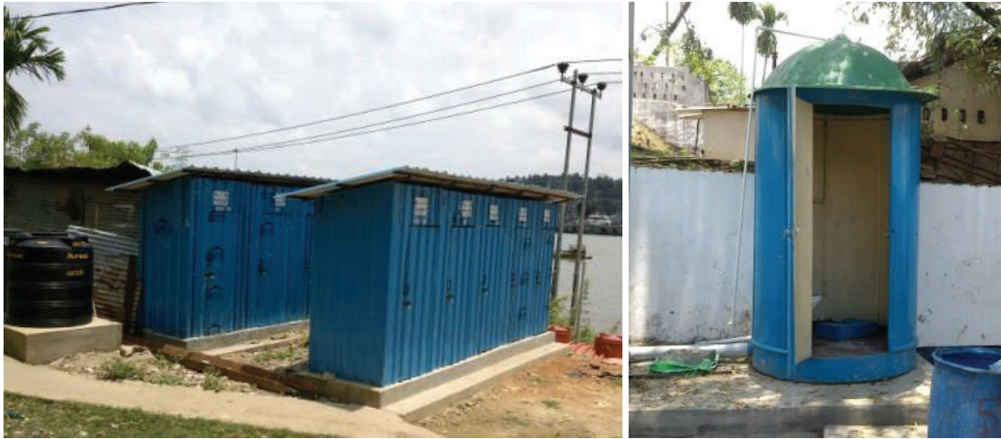
FIGURE 5: NEWLY CONSTRUCTED CT (WARD 7) AND PT (WARD 9) UNDER SBM
