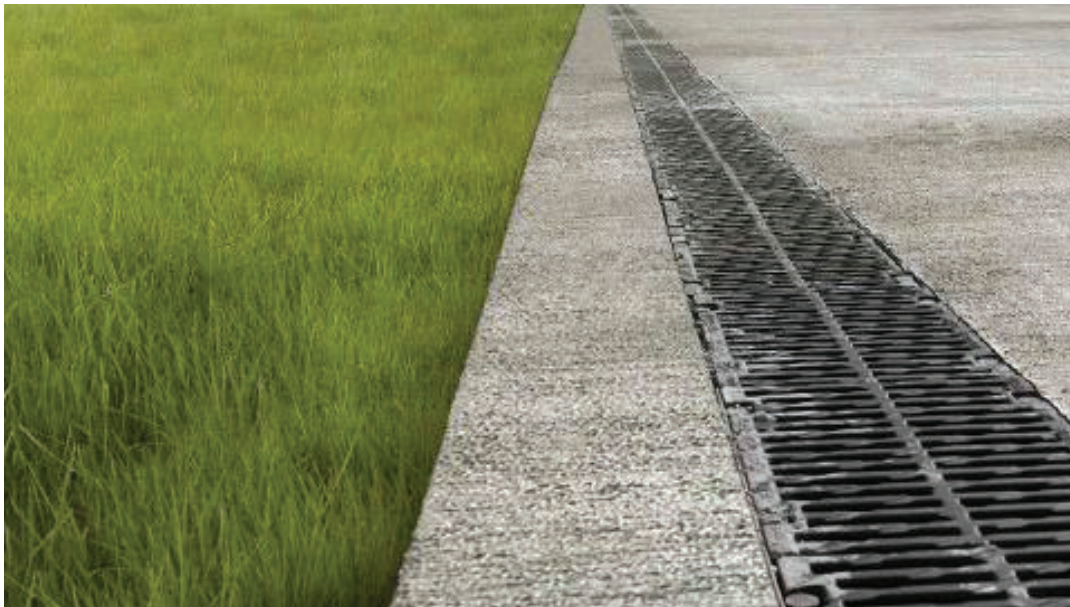
FIGURE 36: SCHEMATIC REPRESENTATION OF STORM WATER DRAIN ALONG THE RING ROAD
