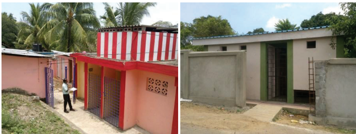
FIGURE 6: UPGRADED AND NEWLY CONSTRUCTED CT (WARD 20, 18) UNDER SBM
