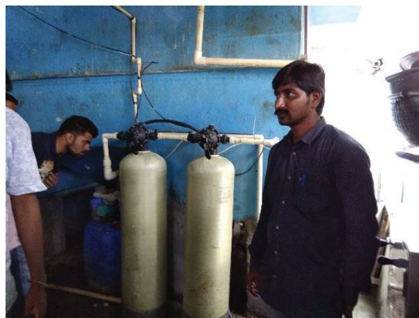
FIGURE 7: CONSULTATION WITH SEA SHELL RESORT AND VISIT TO STP (SBR TECHNOLOGY)
